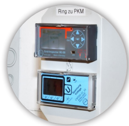
IKI-50 + CAPDIS (Directional Fault Detection)
